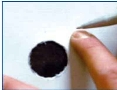
Mark the 6 mounting holes.
