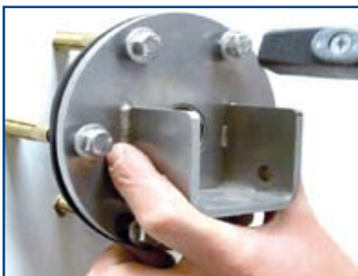
Position the motor flange and drive in the bolts until they are flush with the flange.
