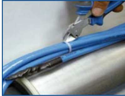
Cut the cable loose with wire cutters.
