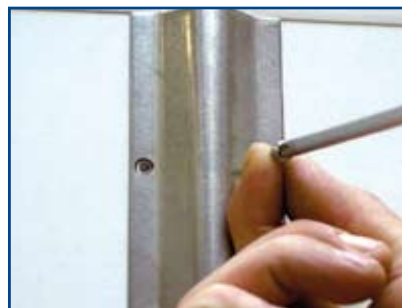
Screw the cable conduit securely in place.
