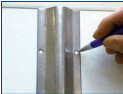
Mark the mounting holes and drill them.
