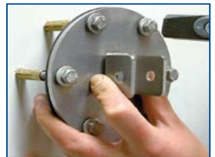
Position the bearing flange and drive in the bolts until they are flush with the flange.
