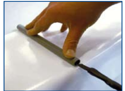
Install an electrical conduit through which the cable can pass under the coping (so the motor can be replaced in the future if necessary).
