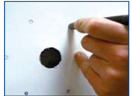
Cut through the liner with an 8 mm punch.
