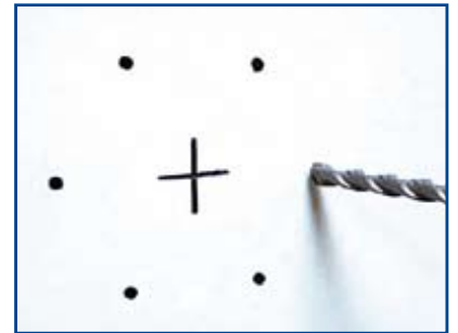
Drill holes with 11 mm bit. At least 80 mm deep.
