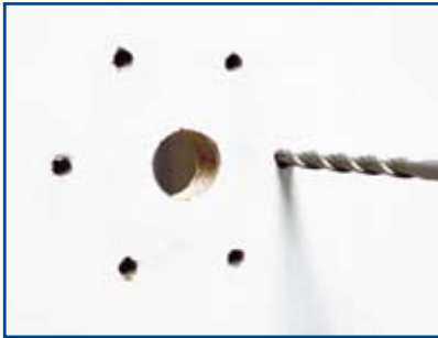
Drill holes with 11 mm bit. At least 80 mm deep.
